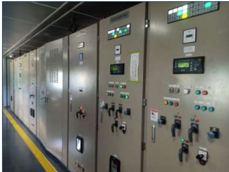
Medium Voltage Switchgear
