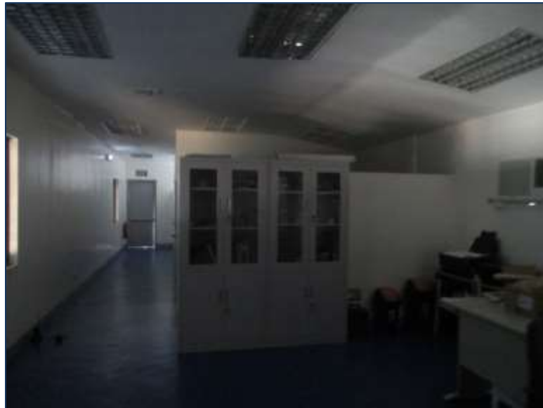
Powerhouse Interior View (Mezzanine Floor)
