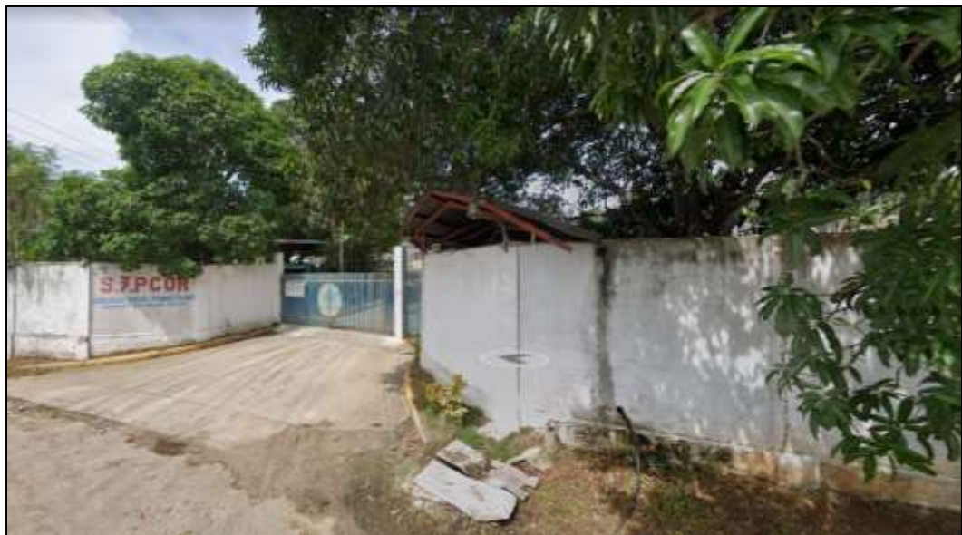
Figure 1: Siquijor Island Power Corporation (SIPCOR) 1 – Siquijor
