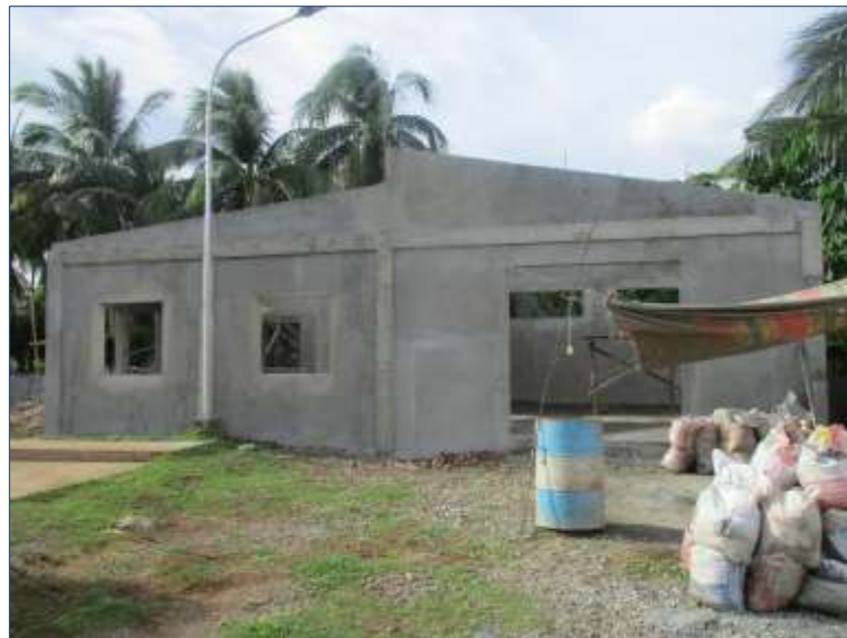
Admin Office Building (Under Construction)
