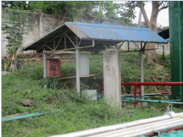
Fire Pump Shed
