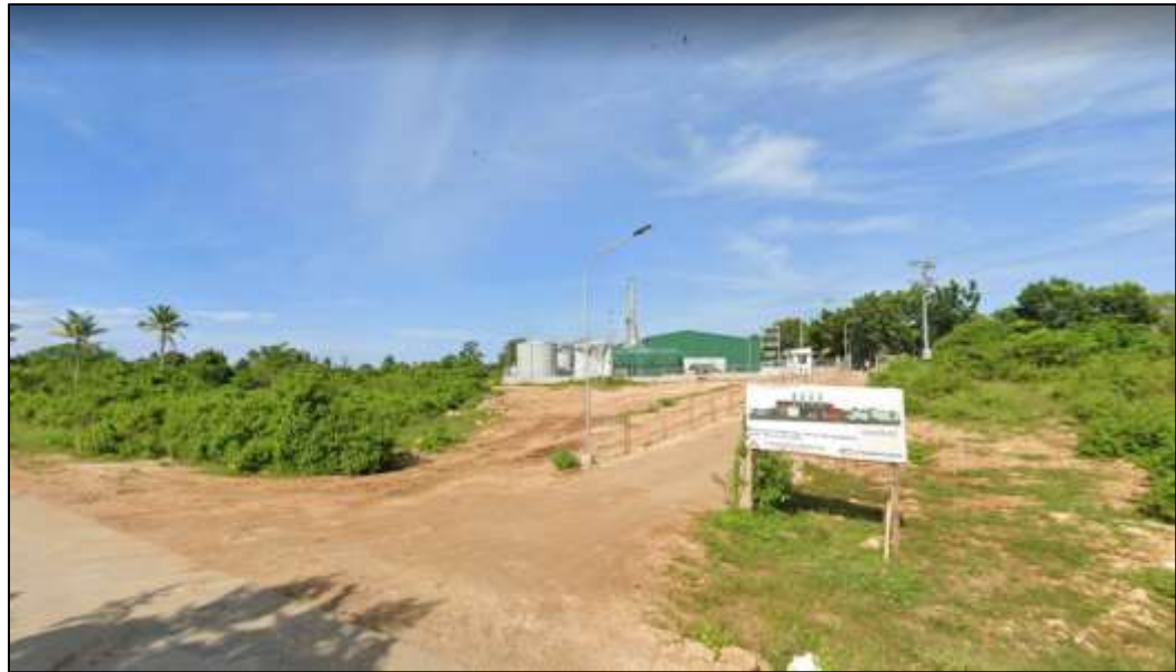
Figure 3: Camotes Island Power Generation Corporation (CAMPCOR) – Poro
