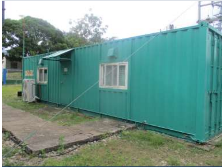
Control Room (Electrical Unit)
